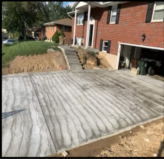
TIGER STRIPES - LOW PRESSURE OR CLOGGED SPRAYER TIP
